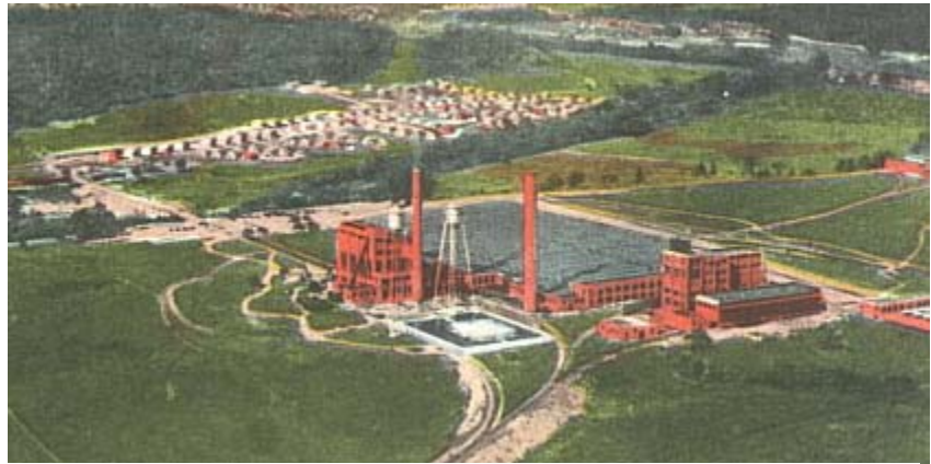
Former International Rayon Corporation's plant built in the 1920.s
